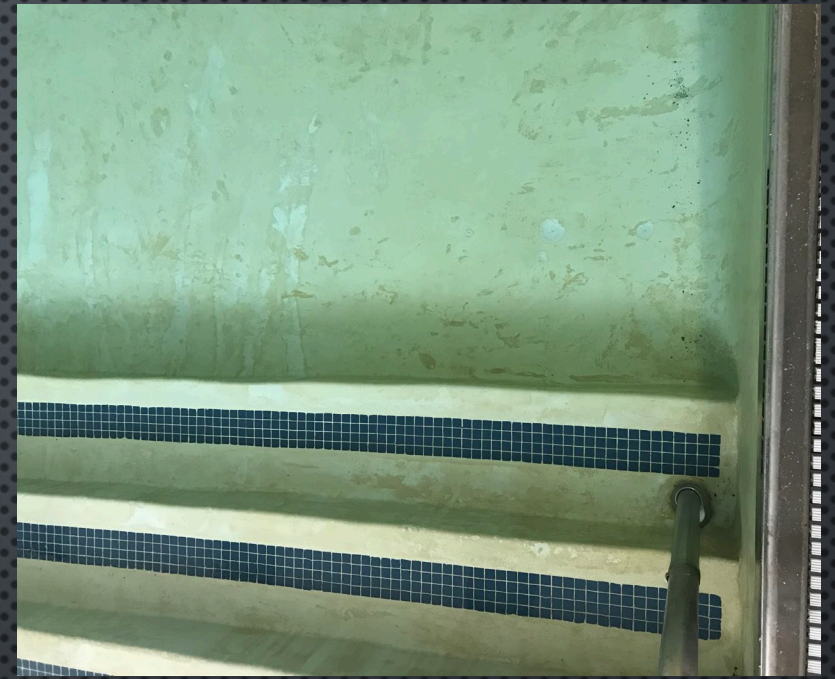
POOL FINISH DETERIORATION
